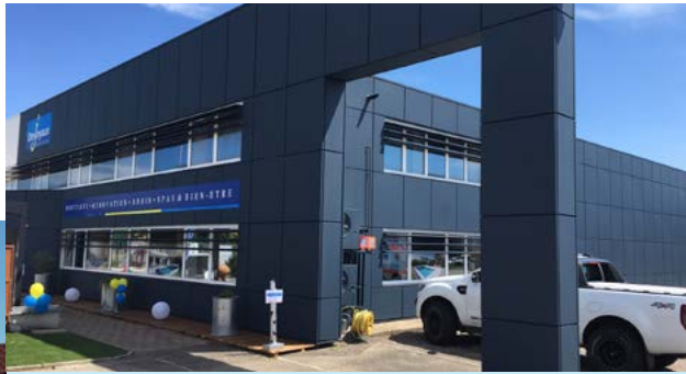
Colmar store renovation.
