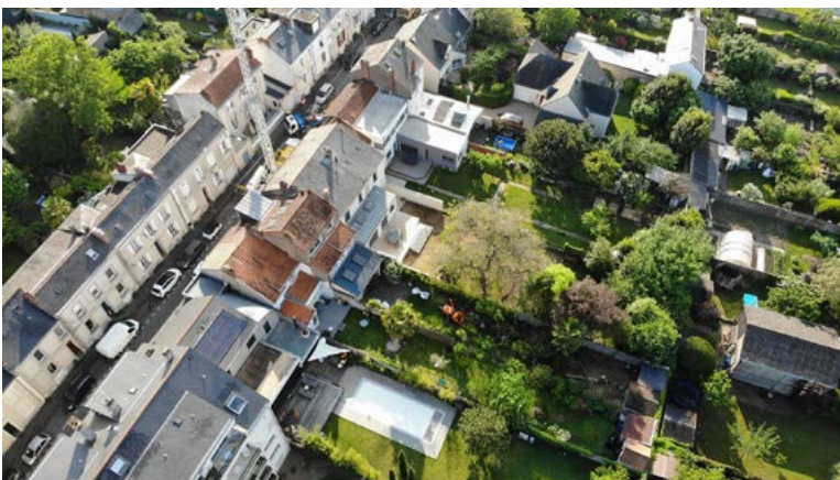
Extensive work carried out by PCREA
