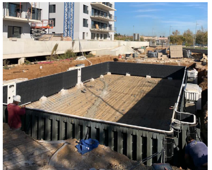
A pool being built in Girona, Spain.
