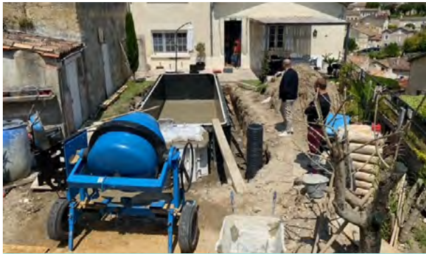
Work in progress in Saint-Emillion by CD Piscines.
