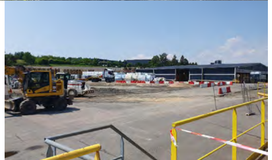
Completion of works for the new reception bays at our headquarters.
