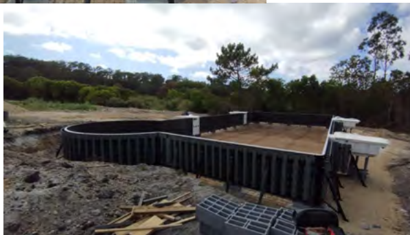
Work on an 18x8 m swimming pool for a Huttopia campsite in Obidos by our Portuguese partner.
