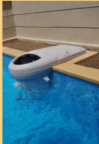
Straddle filtration unit (GR.I 110)
