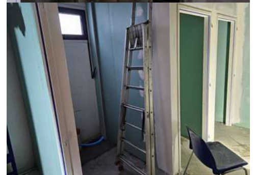
New changing rooms and refectory in Damafor.
