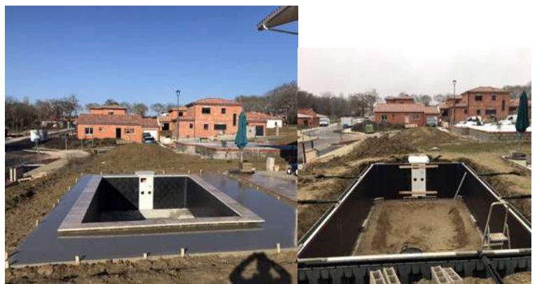
Works underway for SPG Piscines by Ms Gatti in Fenouillet (Haute-Garonne).
