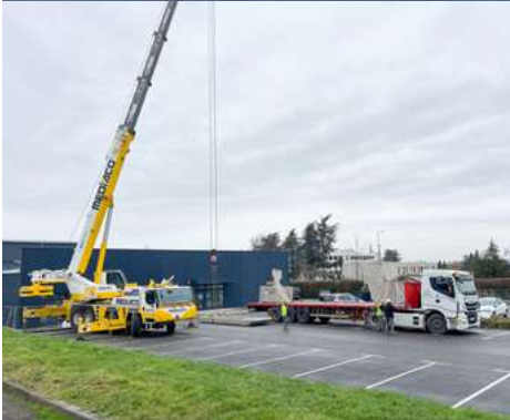
Delivery and unloading of stairs for the new refectory.
